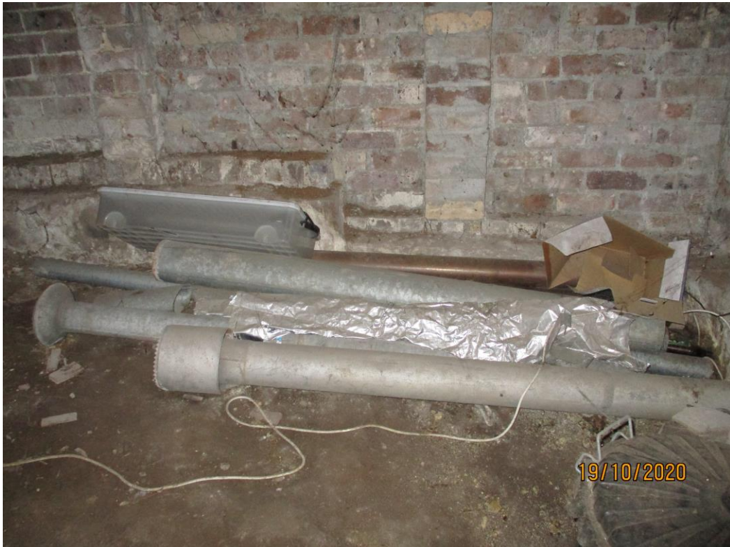
7. Significant amount of debris in the subfloor which will need to be removed
